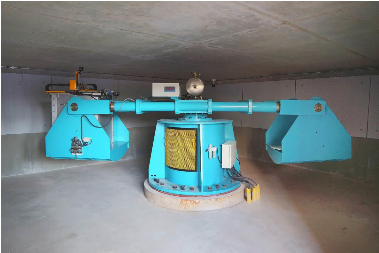
KMITL Geotechnical Centrifuge Facility in Bangkok, Thailand
