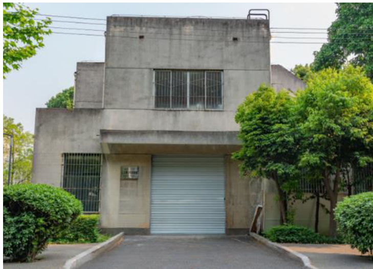
Advanced Geotechnical Centrifuge Test Center.
