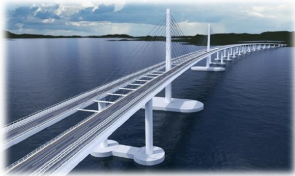
Norway E-39 floating bridge foundation ( www.globalmaritime.com )
